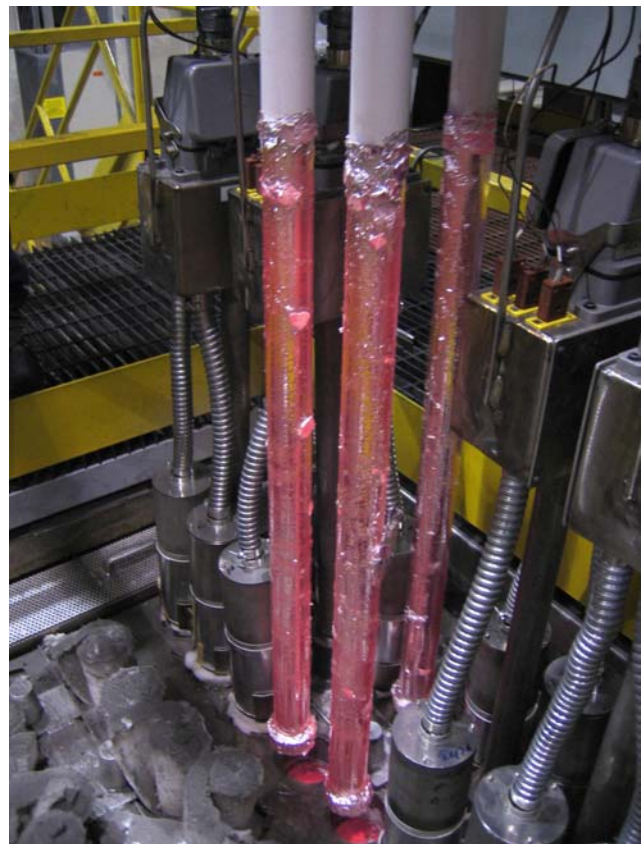
Direct immersion heaters work in a 5,000 lb./hr. ITM. The heaters have a maximum output of 30 kW each.
