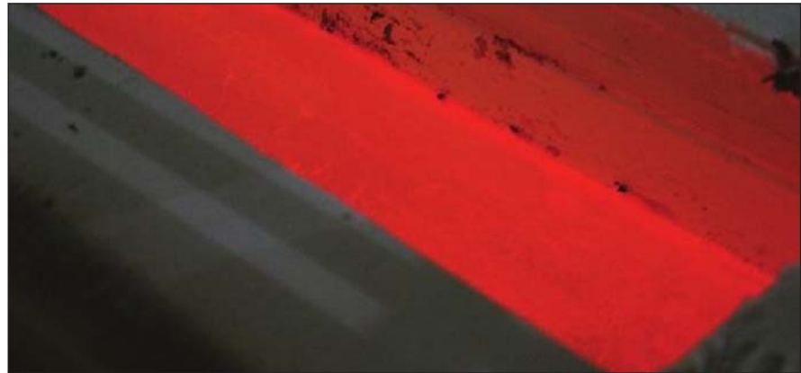
Figs. 1a and 1b. Metalcasting facilities can utilize a combination conductive trough with an integral baffle side pocket panel-heated dip-out well in their melt department.
